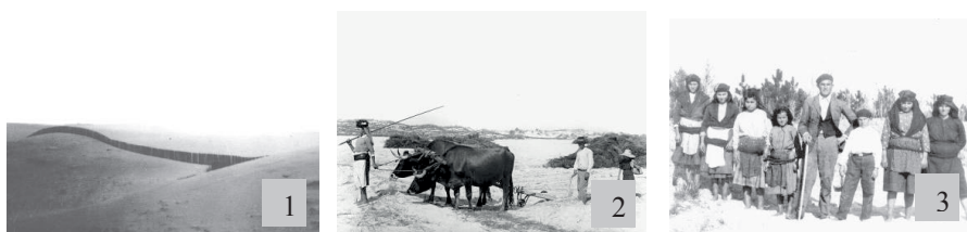
Fig. 1 II- Seeding Dunes 1 - protective barrier: palisade to fix the dunes, 2 -Opening of gullies of sowing; 3 - Family workers in forest sowing
